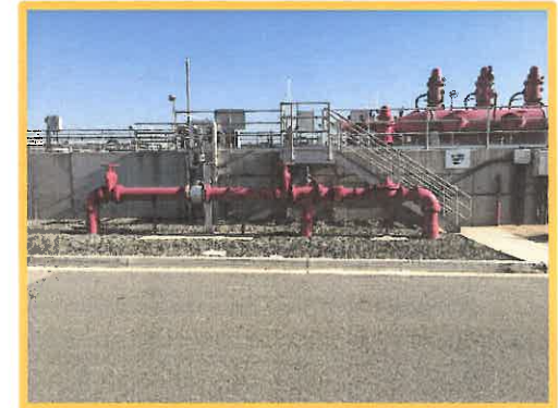
Pump Station Area
