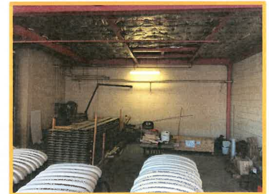
Existing Paint Room
