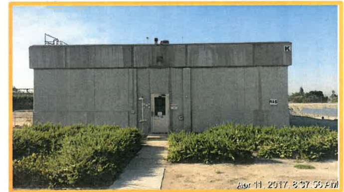
RAS Pump Station Building
