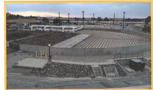
RP-1 Biofilter/Trickling Filter
