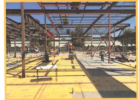
Lab Building Structure
