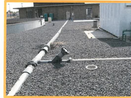
Existing Line at RP-1
