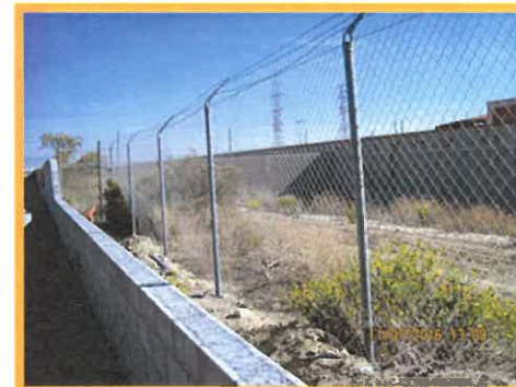
RP-4 Wall to be Completed
