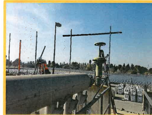
Aeration Basin New Conduit Installation
