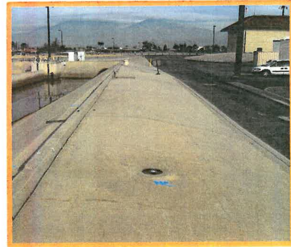
Wash Water Basin Wall to be Modified
