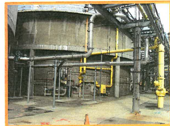
Bottleneck at Digester Area
