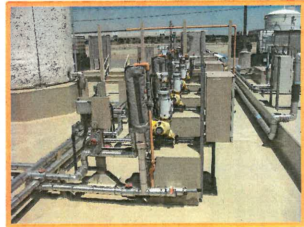
Replace Existing SHS Pumps
