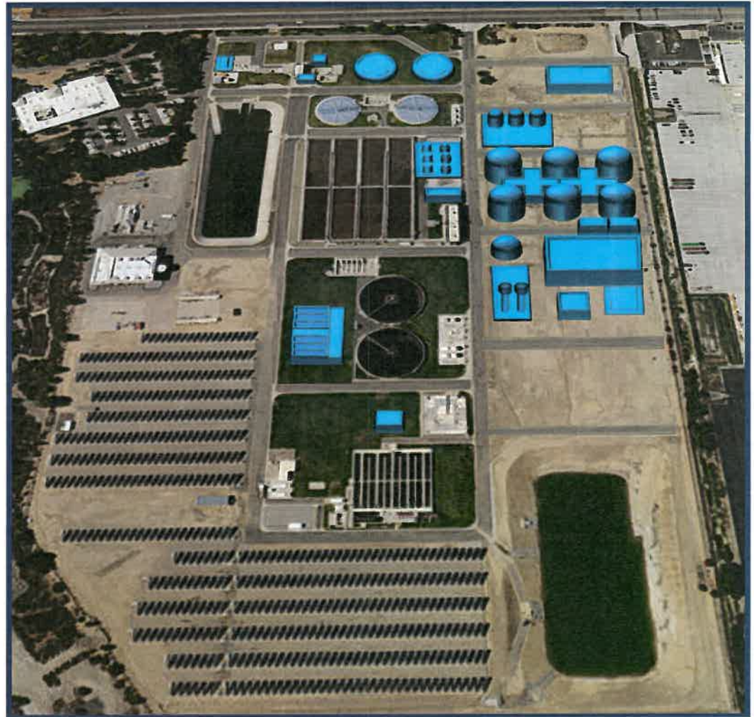
RP-5 Liquids & Solids Treatment Systems
