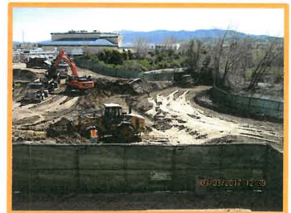
Retaining Wall Area Grading
