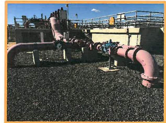
Bottleneck Upgrade Area
