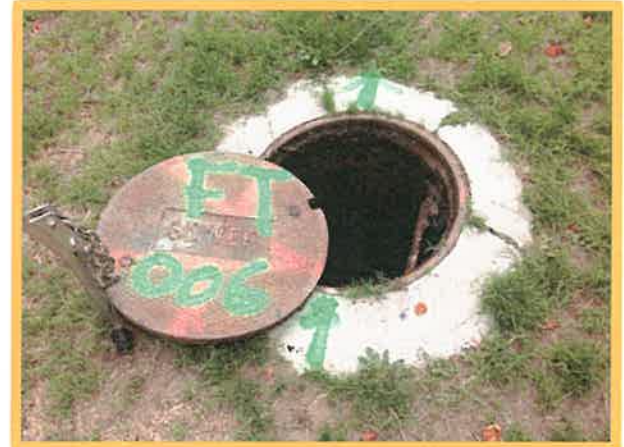
Existing Sewer Manhole in the City of Ontario
