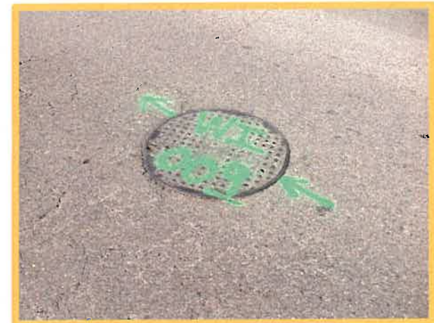
Existing Sewer Manhole in the City of Chino
