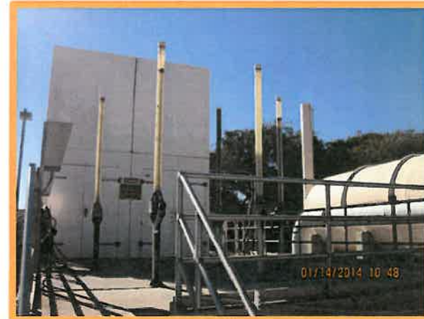
Existing Headworks Structure
