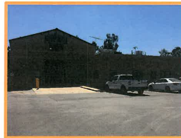
RP-1 Maintenance Bay
