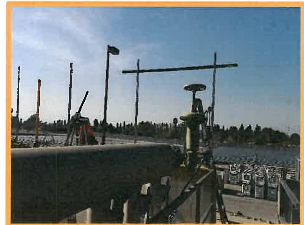
Aeration Basin New Conduit Installation
