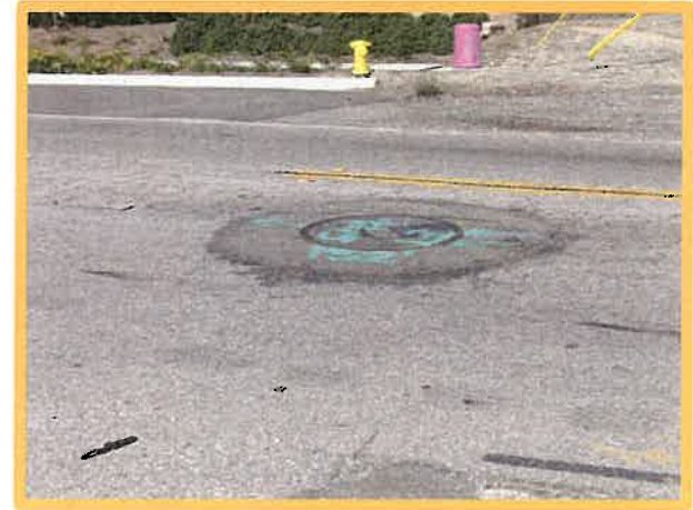
Existing NRW Manhole in San Bernardino County
