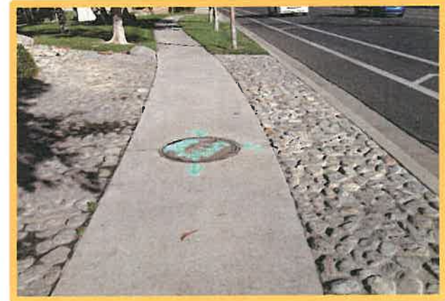
Existing NRW Manhole in the City of Ontario
