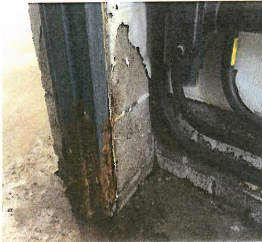
Corrosion Damage
