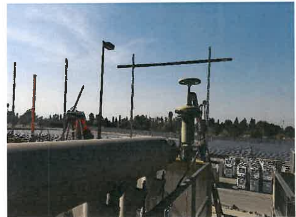
Aeration Basin New Conduit Installation
