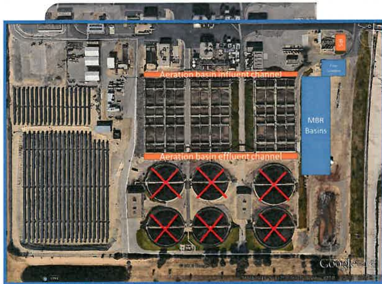
RP-1 Secondary Treatment System
