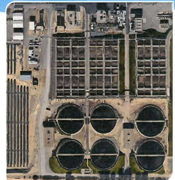
RP-1 Secondary Treatment System
