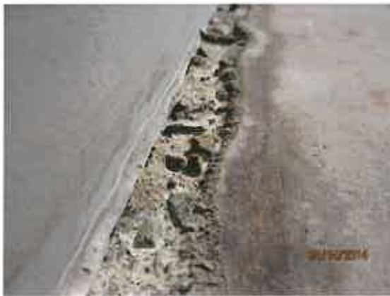
RP-4 Primary Influent Diversion Structure Deterioration
