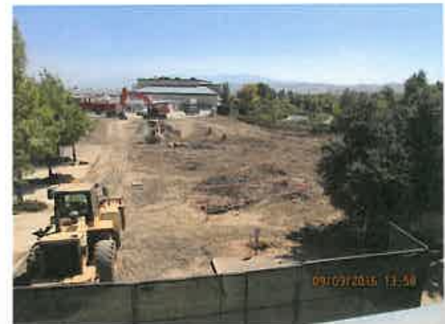
Partial Site Demolition (after)
