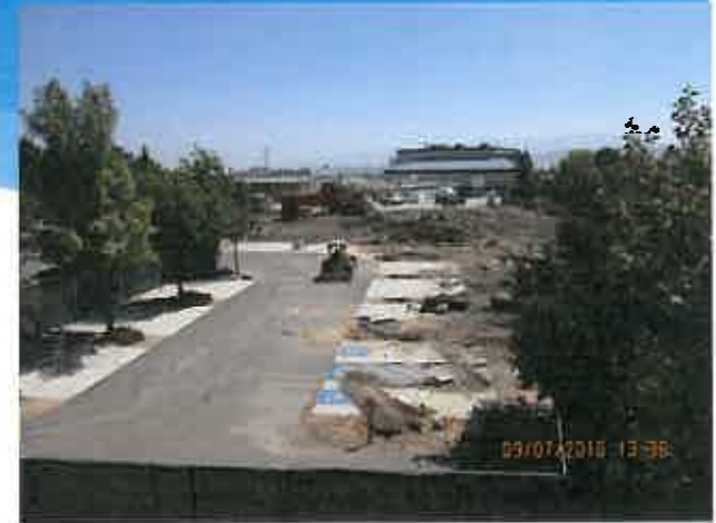
Partial Site Demolition (before)
