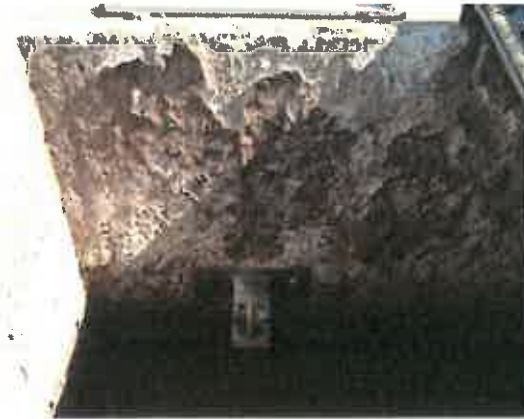
RP-4 Primary Influent Diversion Structure Deterioration
