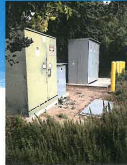
Project Location Behind HQB
