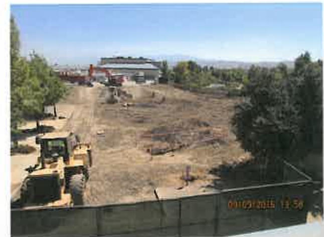
Partial Site Demolition (after)
