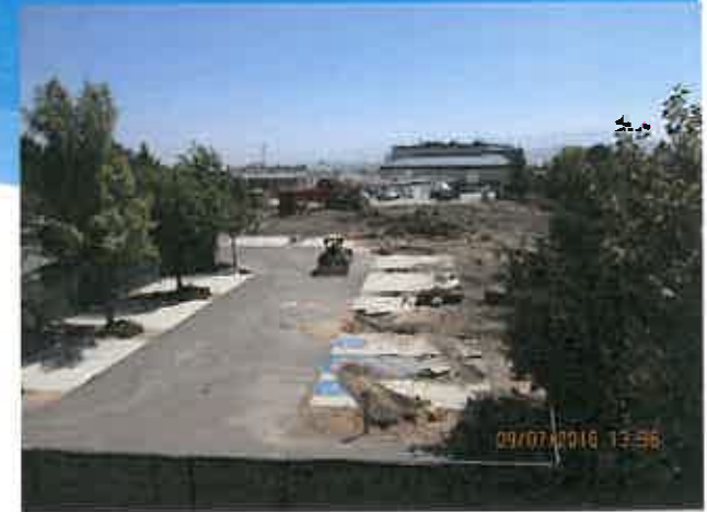
Partial Site Demolition (before)
