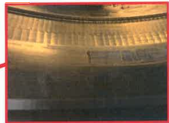
Close up of bearing housing surface damage
