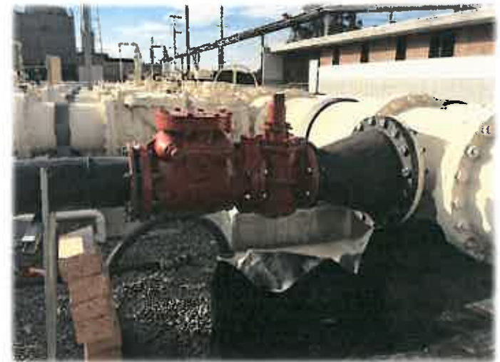
Temporary sewer bypass at SBLs
