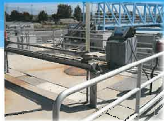
Primary Effluent Diversion Structure
