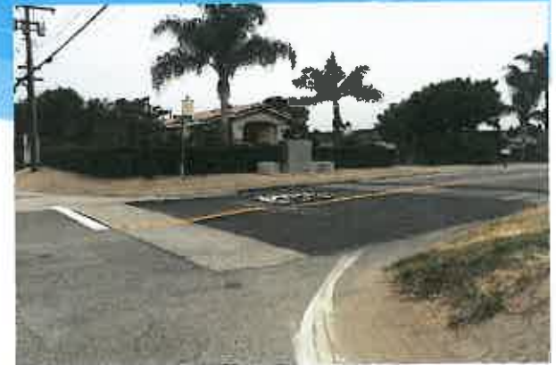
New Control Panel Installed & Street Paved
