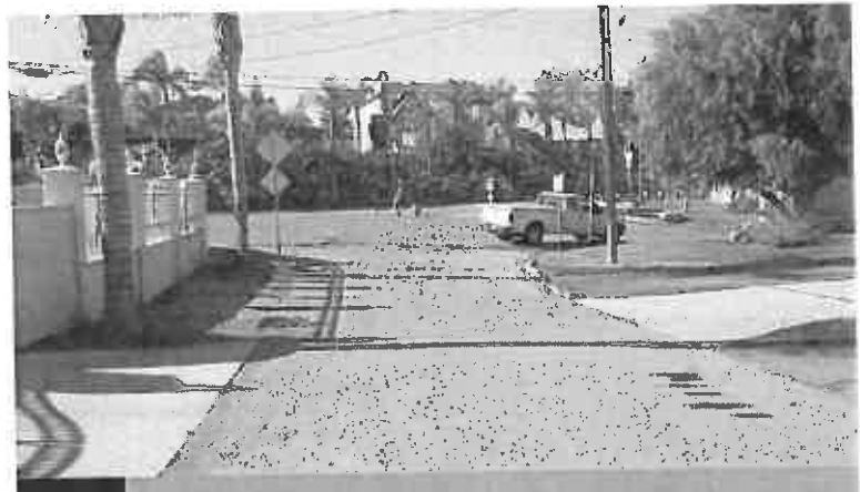
8 Proposed site for installation of pipeline reconnections at Lolita Street and Santiago Canyon Road
