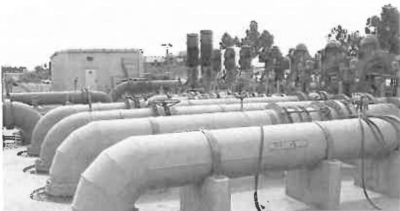
RP-1 Recycled Water Pump Station discharge pipelines
