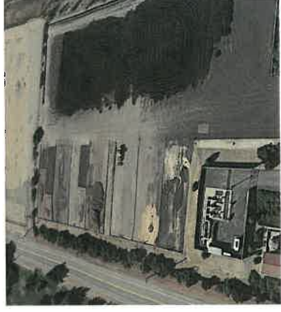
RP-2 Sludge and Solar Drying Beds
