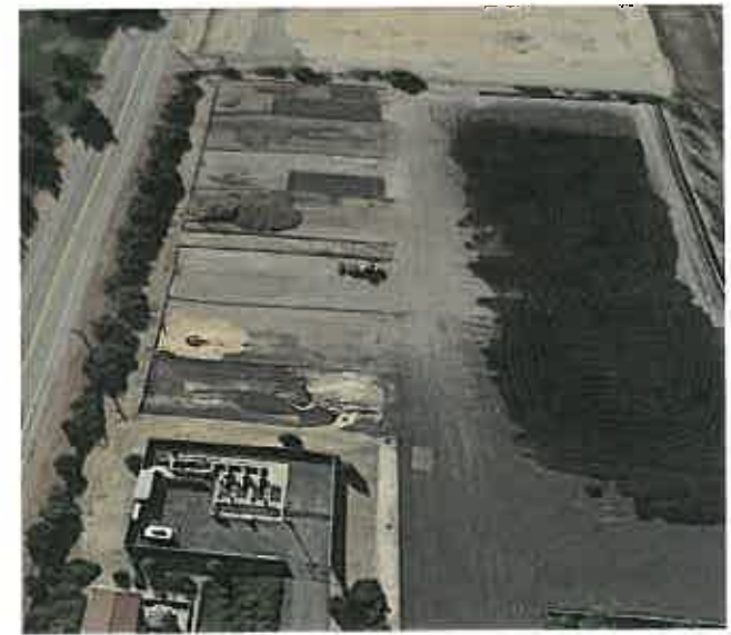
RP-2 Sludge and Solar Drying Beds
