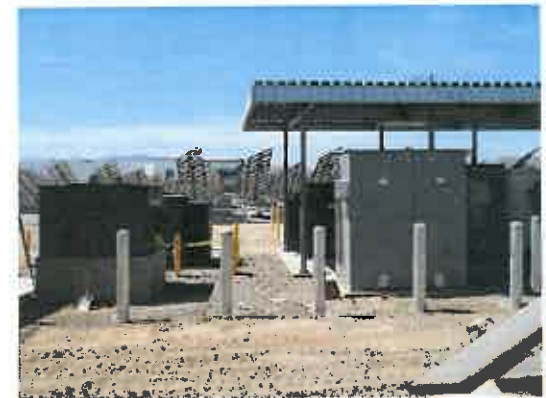
PME and Solar NGOM Installation
