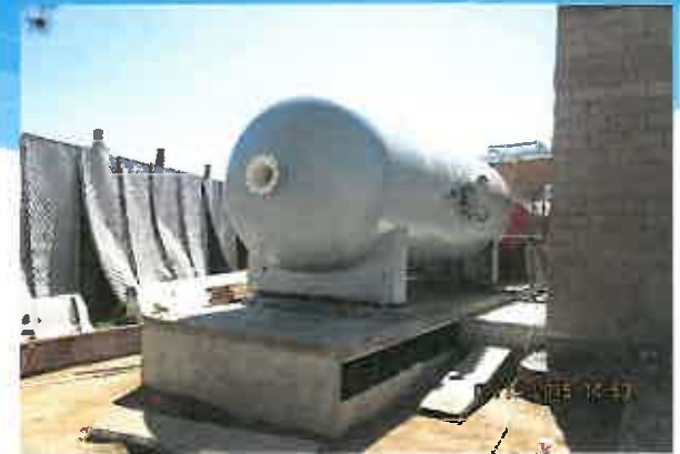
Surge Tank Installed on Pad
