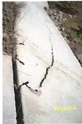
Concrete Displaced By Water
