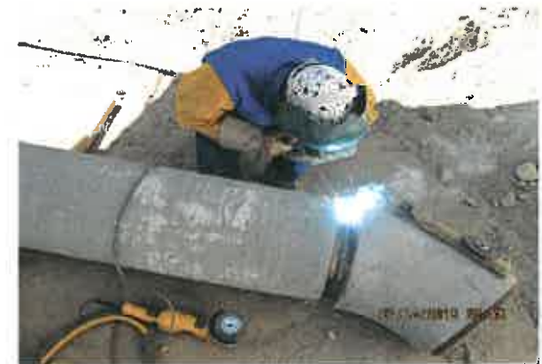
Welding 12-in RW Pipe
