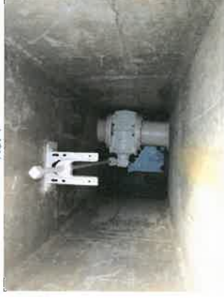
One of two 18" valves in DAF Valve Vault No. 1
