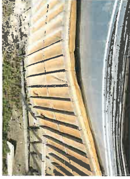
Aeration Panel Membrane & Base Plate
