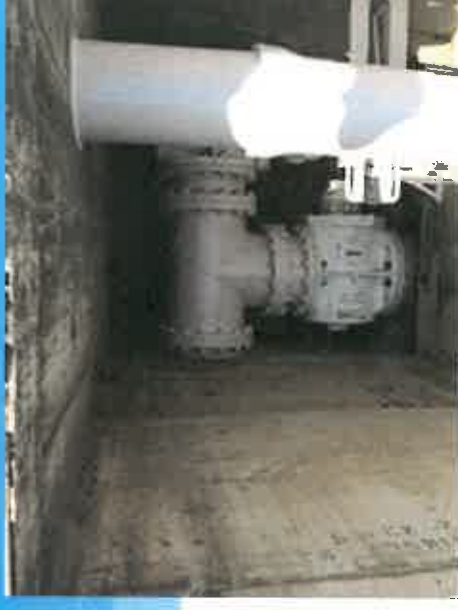
One of two 18" valves in DAF Valve Vault No. 1
