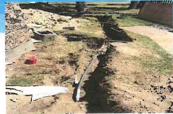
Relocating Existing Utilities
