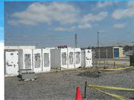
Tesla Powerpack Units
