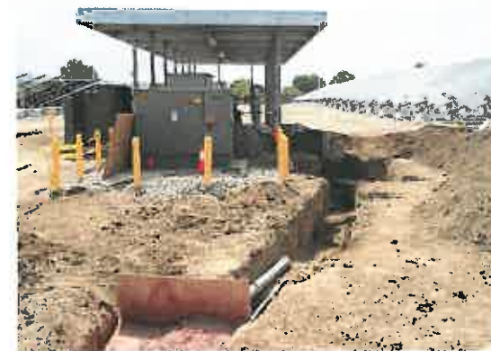
PME and Solar NGOM Installation
