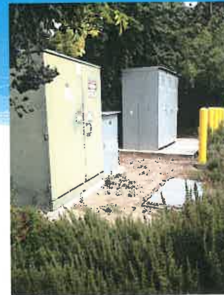
Project Location Behind HQB
