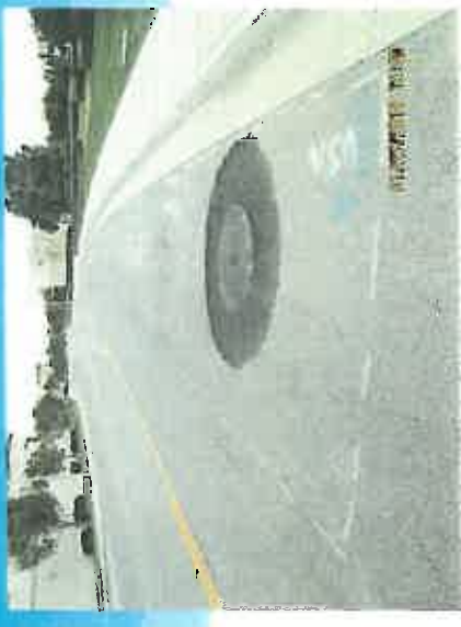
Manhole Adjustment Complete
