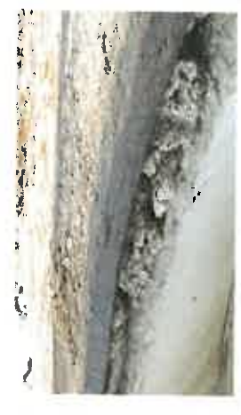
Deteriorated Grout
