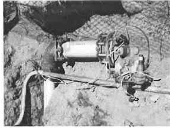
Vineyard Elementary RW Pipe Replacement
