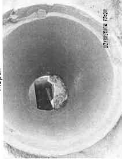
RP-1 42-inch Primary Effluent Pipe Repair
