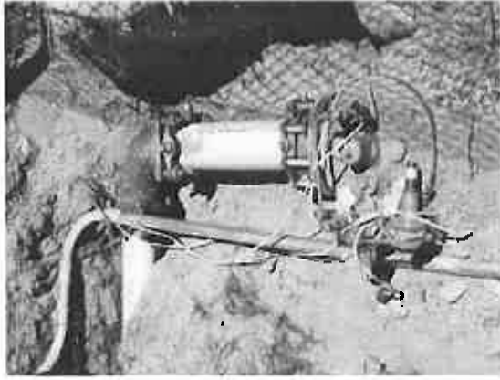
Vineyard Elementary RW Pipe Replacement
