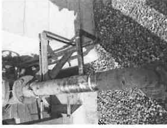
Potable Water Line Installation at RP-4
