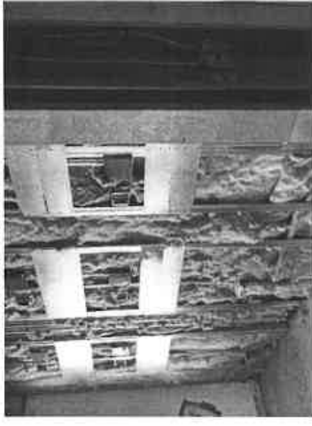
Control Room Wall Modifications
