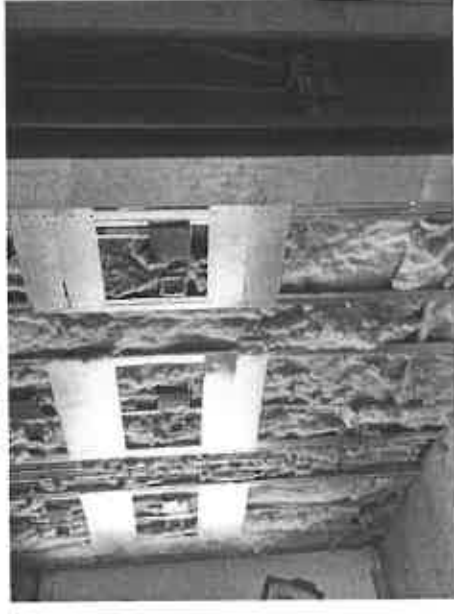
Control Room Wall Modifications
