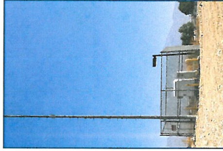
Montclair Basin Tower
