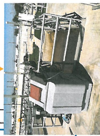
Secondary Clarifier Splitter Box
